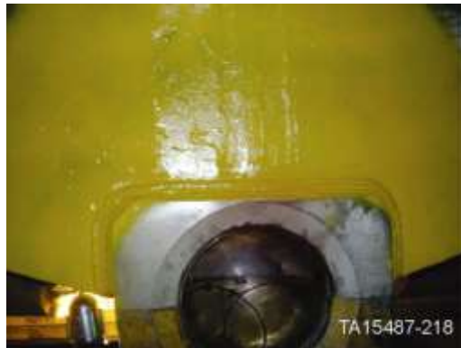
Paint the weld repair area
