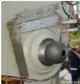
Typical ceramic heater locations on outside of frame
