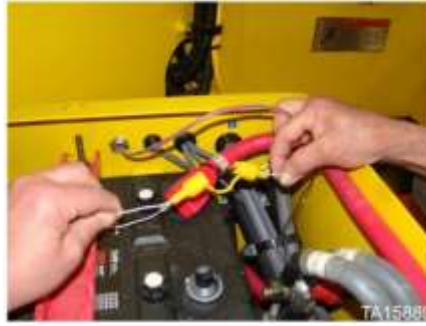
Fire suppression in-line fuse located in loader battery box on some machines
