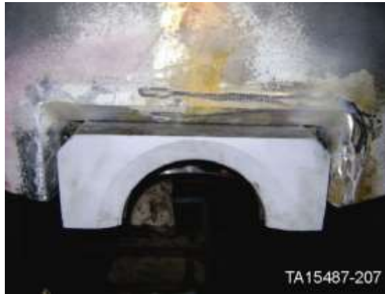
Socket tack welded in place
